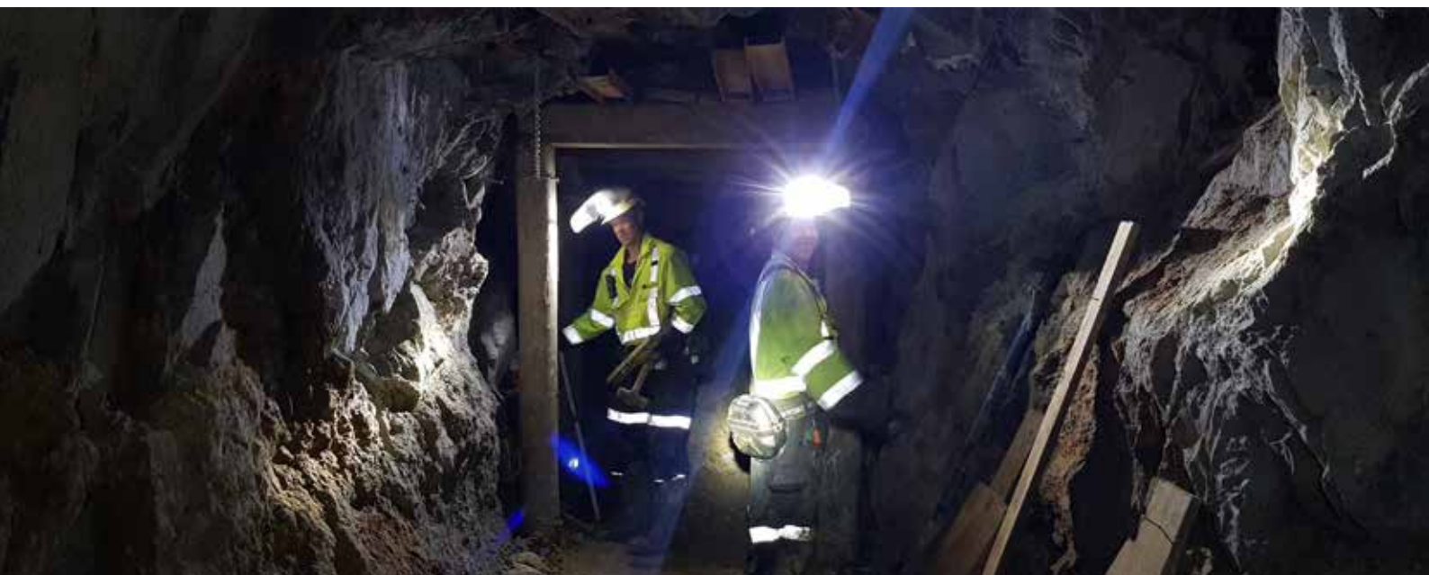
Timber sets being constructed to reinforce the brow at the entrance to the Dubbo Rise
