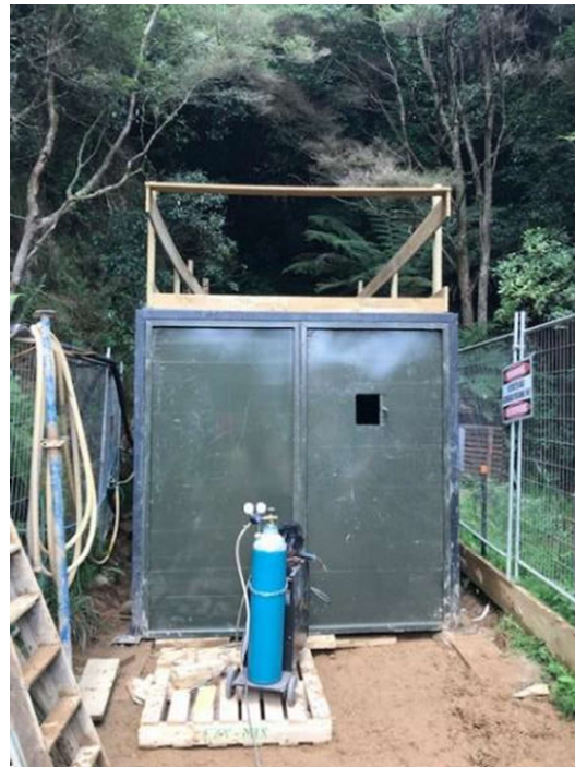
Figure 2 - Completed ventilation lock at No 8 Level Portal
