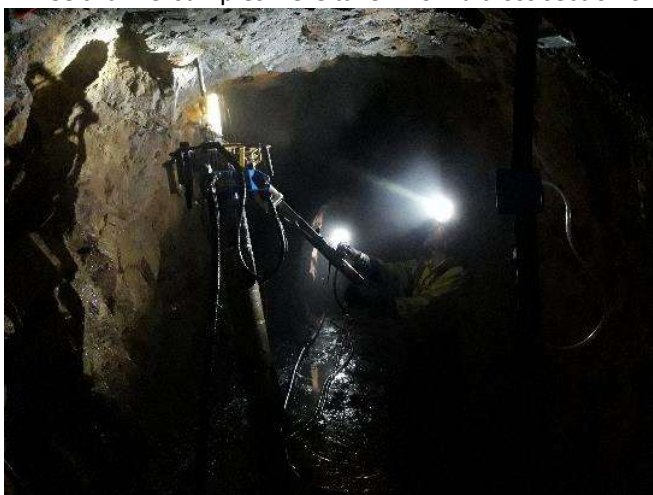
Figure 3 - installation of rock bolts in Keillors Crosscut
